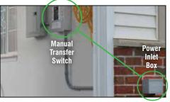
**30 Amp Outlet & Manual Transfer Switch** Allows generator to be easily connected to a permanently installed manual transfer switch to power several circuits and hardwired appliances such as a furnace or sump pump.
